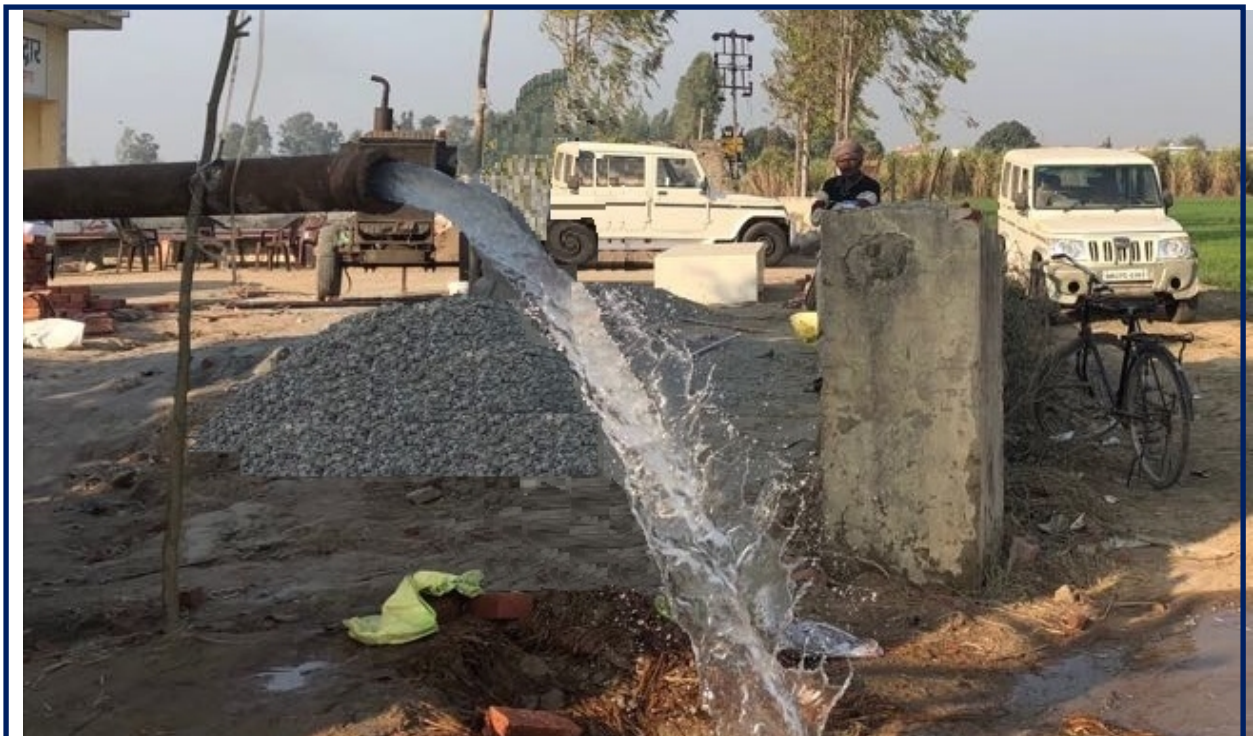
Figure-5: Well # F, Near Kurukshetra under Development Stage
